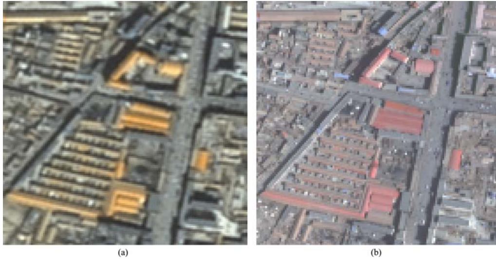
Fig. 5 Remote sensing images of the brick building before (a) and after (b) the earthquake
